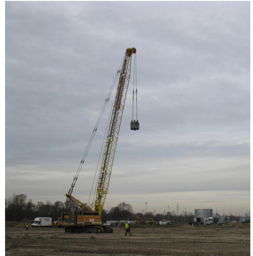
Fig. 18. Dynamic compaction in Gdansk Menard Group.
