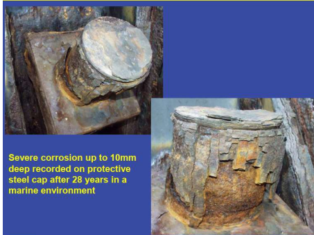
Severe corrosion and deterioration of bitumen painted steel cap after 30 years in service
