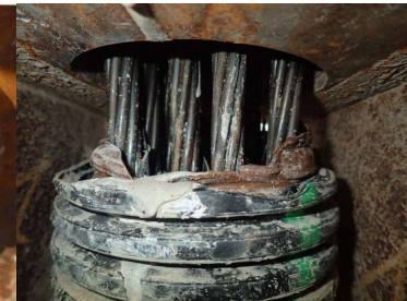
Removal of protective cap reveals severely corroded barrel and wedges after 11 years in service
