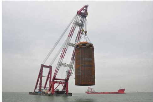
Hong Kong-Zhuhai-Macau Bridge, d~20 m, L~40 m, m=600 t
